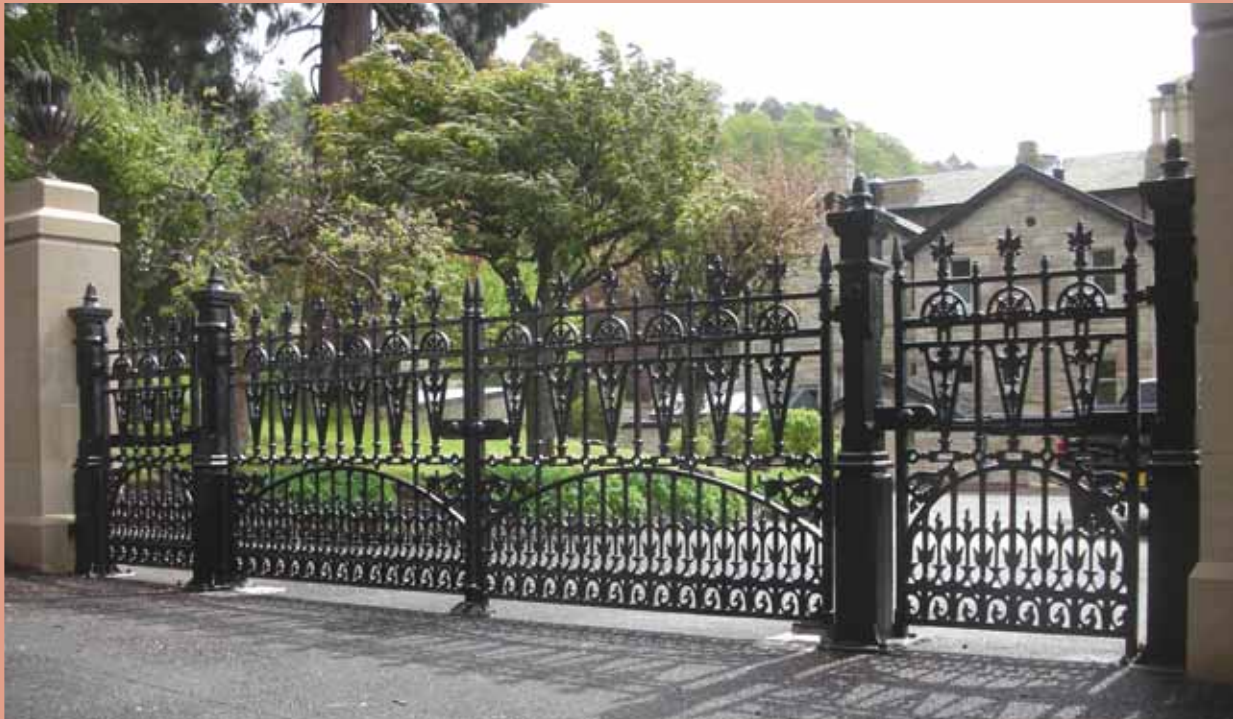
Gilberton driveway (12ft) and pedestrian gates with Pillar posts
