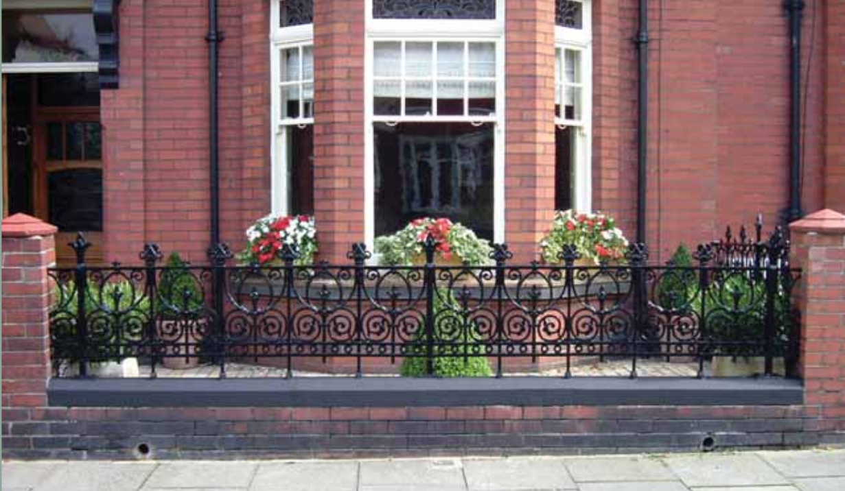
Prospect railings with posts
