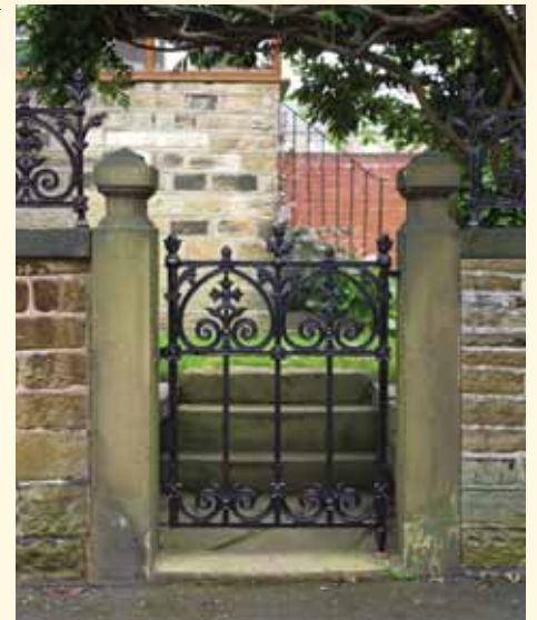
Terrace pedestrian gate with existing stone pillars
