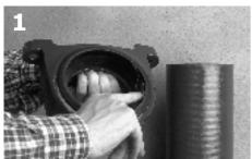
1. Apply a small amount of lubricant (ie lubricant prod. code 199037) on the lip of the rubber gaskets, both ends, to ease insertion of pipe/fittings.
