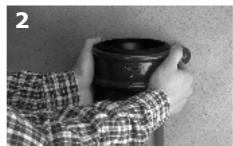
2. Push joint over the end of pipe/fitting, ensuring the central register is abutted against the spigot edge evenly. If the joint is eared, fix to wall using anti-corrosion coach screws or similar.
